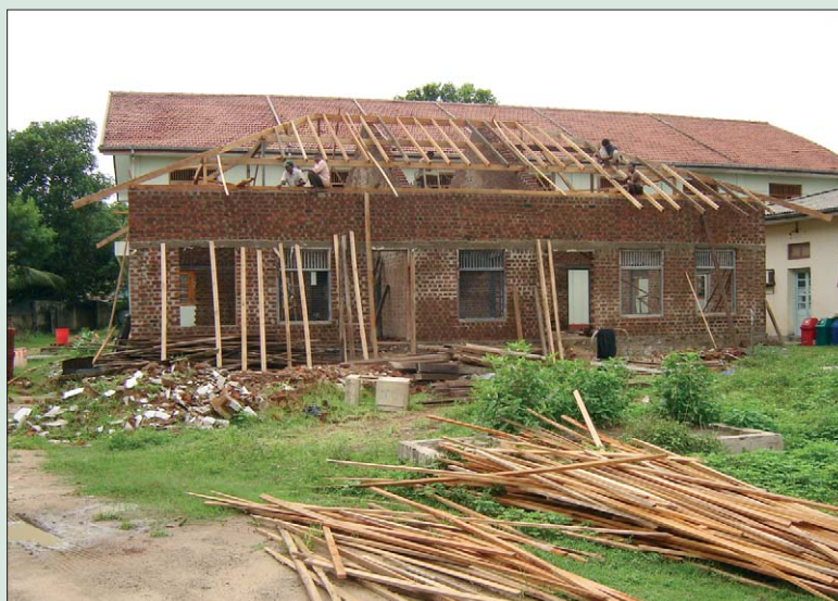
Figure: Construction of a mental health unit in Kalmunai, Sri Lanka
